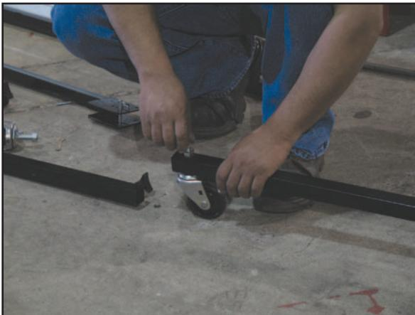
There are 3 holes at the end of each side of the base. Unscrew the nuts on the wheels and insert a wheel on each side of the base. Tighten the screws on the wheels.
