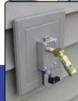
Exterior Mount Air outlet is mounted outdoors
