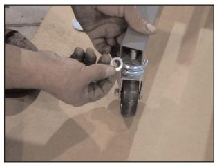
Place locking washer on post of Caster (E) and fully tighten nut. Insert cap from Caster Assembly (E) on end of Main Body (A) post. Repeat on all 4 corners of Main Body.
