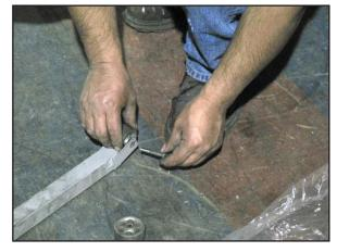
Place the wheels on the back of the base. Insert the bolt and tighten the nut.
