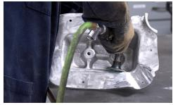
Aggressively sand the inside surface of the aluminum reinforcement plate with 25 to 60 grit sandpaper on a Roloc® disk. Sand every surface that will touch the hood until the sanding scratches have 100% coverage. It's very important to leave no unsanded surface where adhesive will be applied on both the plate and the hood. Hand sanding parts of the reinforcing plate will also be required in this step.
