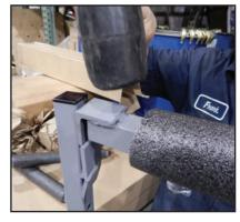
**2.** Using a rubber mallet, gently tap the metal tab of long arm in to the top slot of the wall mounting bracket.
