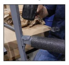
**3.** Repeat this step placing the tab of the short arm in the middle slot of the wall mounting bracket, and the remaining long arm in the bottom slot. Do these 3 steps with both wall brackets.
