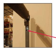
**4.** Level out the wall brackets and screw to the wall. (Screws not included)
