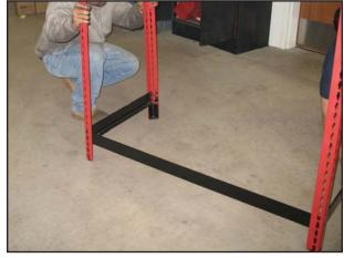
Work your way around the Deluxe Parts Station inserting cross beams into the corner uprights as shown above.
