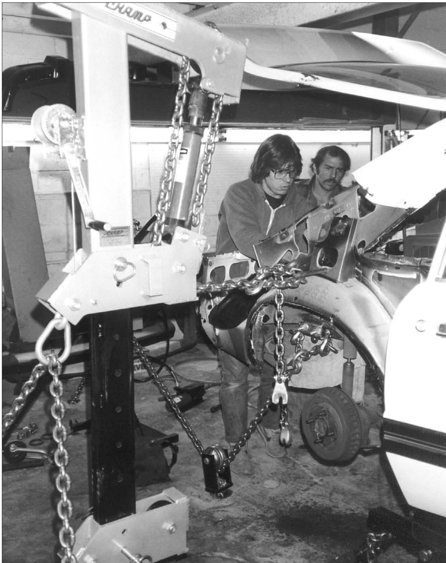
OWNER AND METALMAN EXAMINE PROGRESS OF REPAIR.
