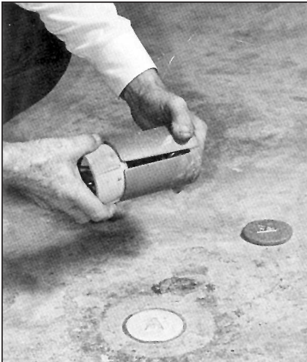
5. Firmly insert anchor expander with chain into anchor sleeve.
