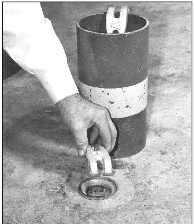
4. With anchor expander dislodged from anchor sleeve, attach puller klaw to protective ring at top of sleeve.
