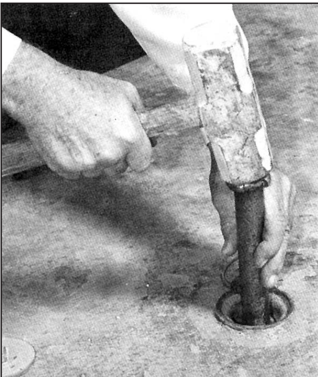
3. Striking a firm hammer blow, dislodge anchor expander from anchor sleeve. Take care not to damage retaining wedge.
