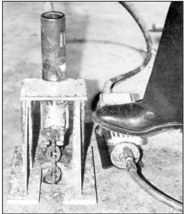
4. With ram fully retracted apply pressure to foot pedal to begin pressing anchor into floor.
