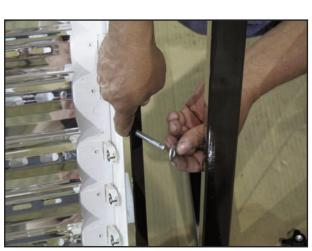
Slide 2" bolt (D) through hole on bracket attached to Light Housing (C). Repeat on both sides of Light Housing (C). *NOTE: washer must be between frame structure and light bracket.*
