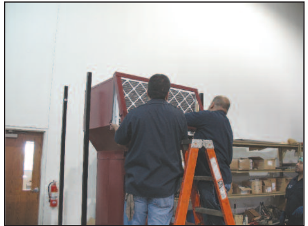
Install two odor ban carbon pleats in front of the exhaust panel filters.
