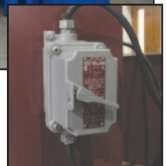
Unit is turned on & off using the switch mounted on the side.
