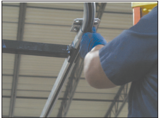
Mounting brackets are already loosely installed on curtain rails. Tighten bolts on brackets to hold rails together.
